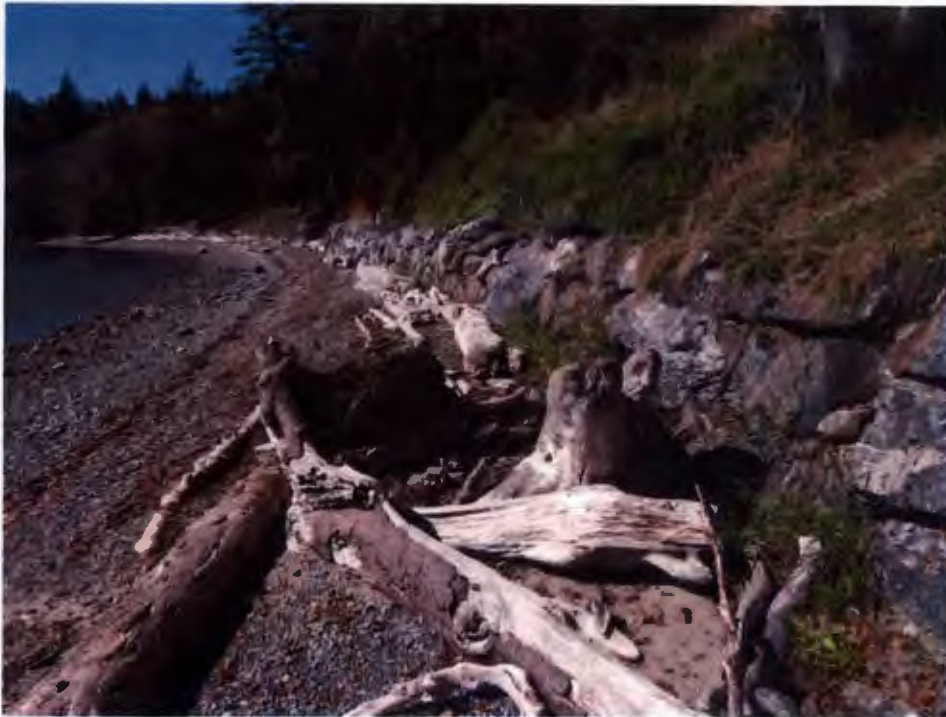
Photograph 5 – New wall east end (2)
