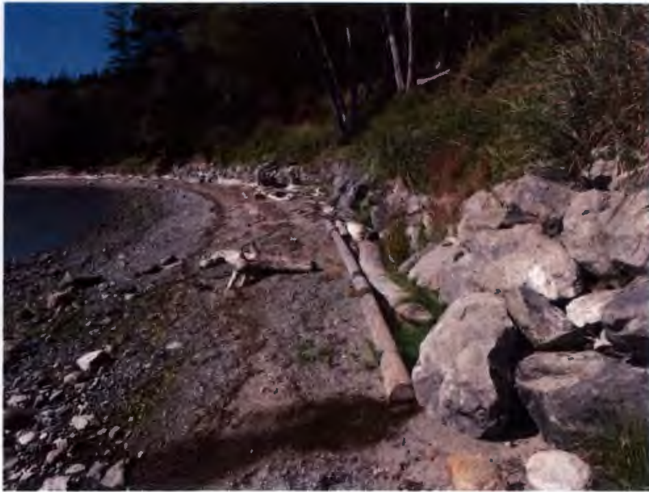
Photograph 3 – Transition from old to new wall (at base of alders)
