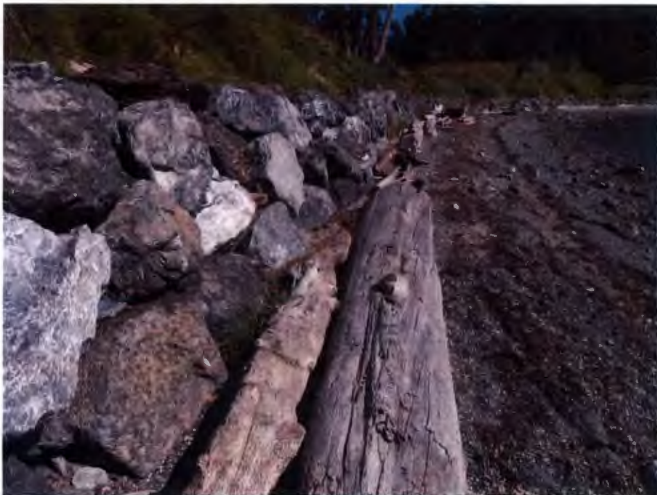
Photograph 6 – New wall center to east
