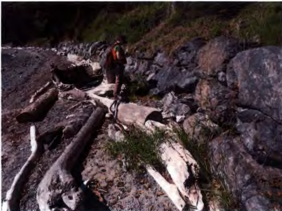
Photograph 4 – New wall east end (1)
