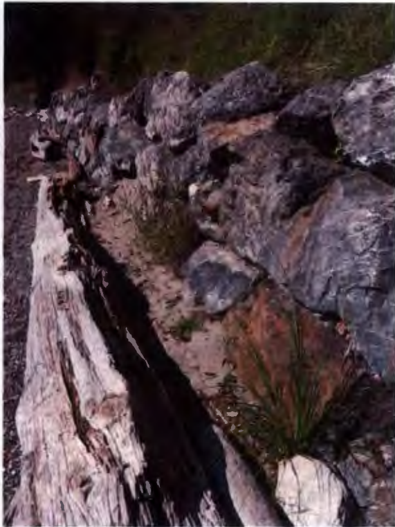
Photograph 7 – New wall center to west
