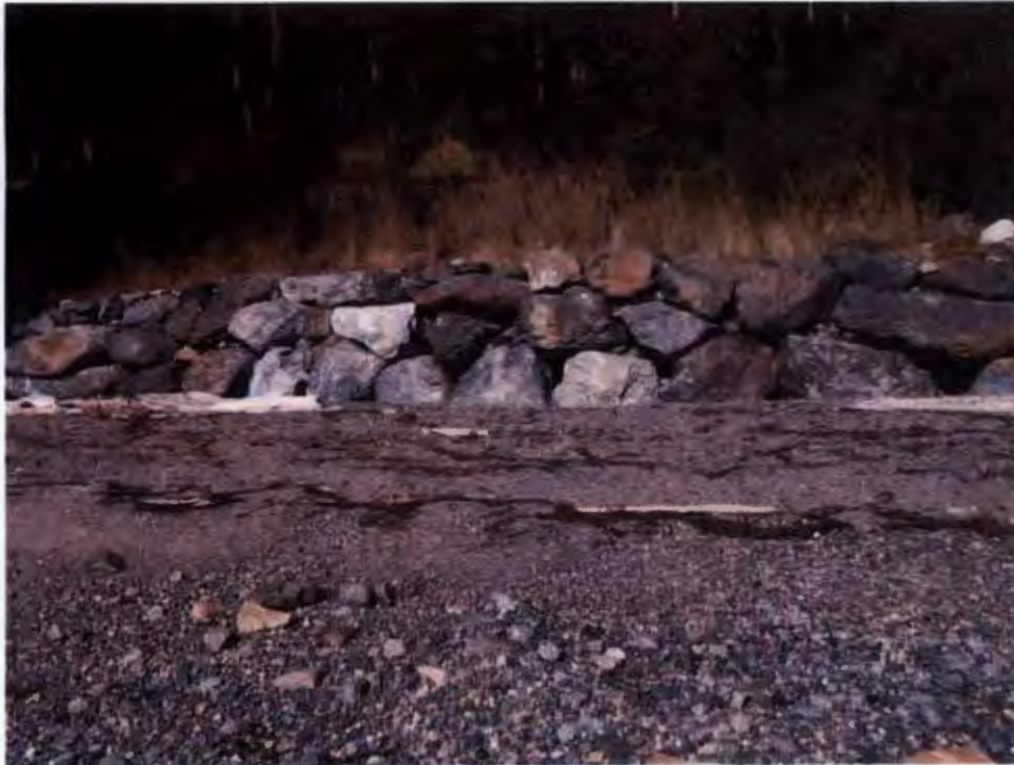
Photograph 12 – Center of new wall
