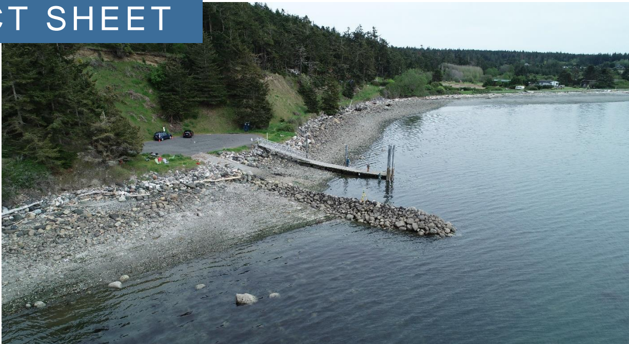
Photo: Mackaye Harbor boat launch - Coastal Geologic Services
