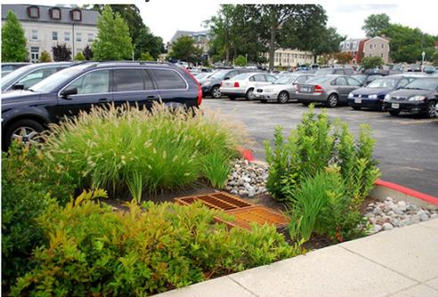
**How we're doing it-** Bioswale and rain garden construction follows the Department of Ecology's BMP construction requirements and design. An engineered compost mixture of organic compost and sand are layered and planted with a variety of native plants and wild grasses to increase biofiltration.
